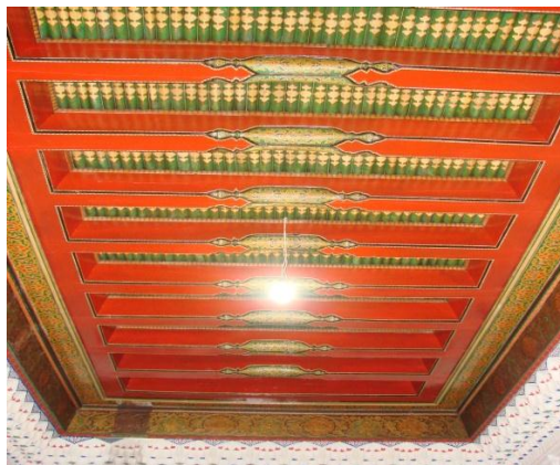
Pic.2. Ceiling of traditional house
