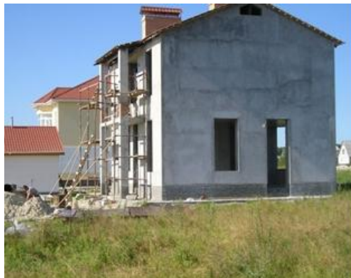
Figure 1 - Residential two-storey house, erected with the use of aerated concrete wall panels
