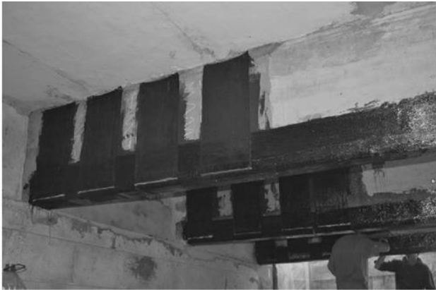
Pic. 2. Repair of reinforced concrete structures using composite materials
